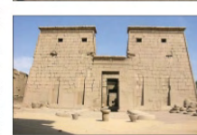
Top: The outside wall of the open court of the Temple of Khonsu (looking west) Bottom: The front of the Temple of Khonsu (looking east)
